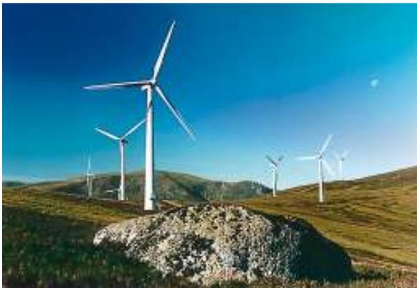
Larger machines are likely to be in much windier areas. Just doubling the wind speed from 4m/s (poor inner city site) to 8m/s (good elevated rural site) would yield 8 times more potential energy output.
